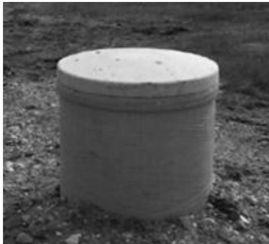
Well lid on a bored well (Photo Credit: Manitoba Water Well Association)
