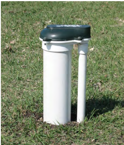
Well cap on a drilled well
