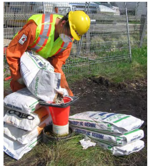
Sealing an abandoned well
