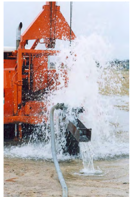
Developing a well by air lifting
