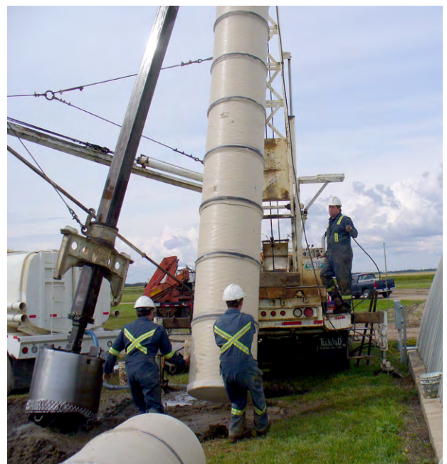
Installing a large diameter well casing
