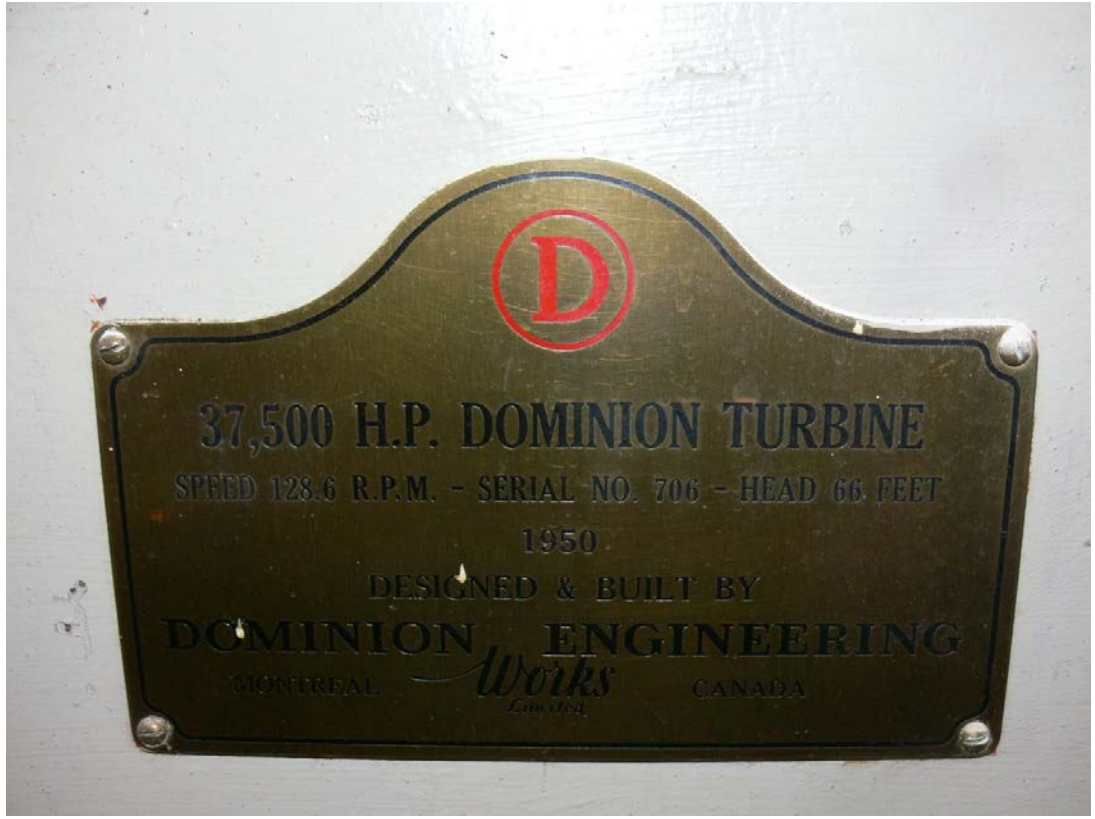
Figure 15 Unit No. 5 Nameplate Original, 1952
