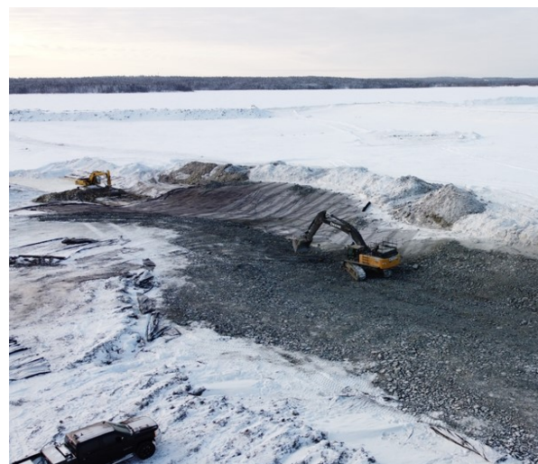
Excavators placing rockfill to stabilize slopes in the tailings management area.
