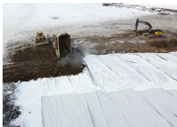
Rock truck and dozer spreading clay fill on a stabilized subgrade
