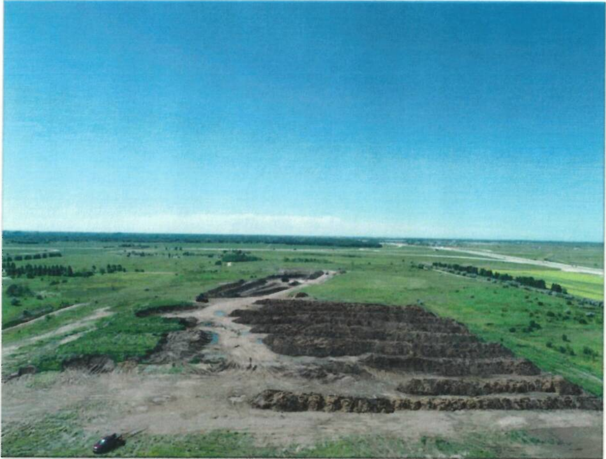
Aerial of Site June 28 th at end of project:
