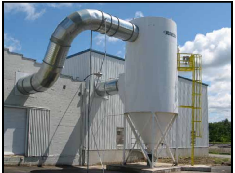
Model 10SWF504 on Paper Dust - Packaging Industry
