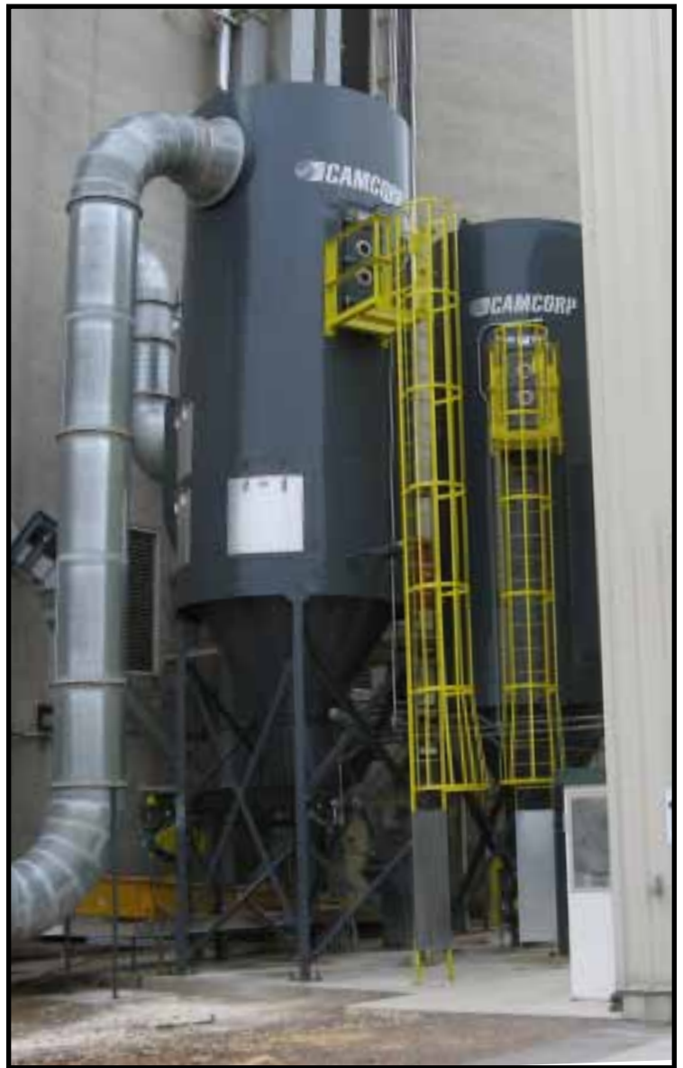
Model 10SWF256 & 10SWF312 on Corn Dust Ethanol Industry
