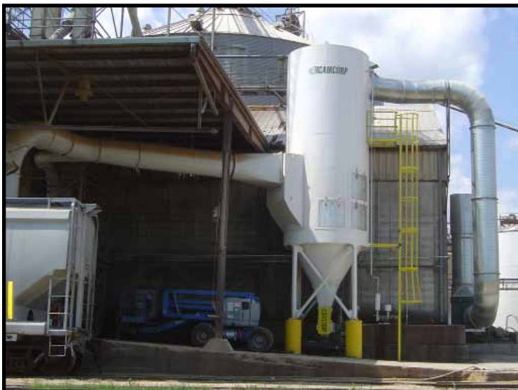
Model 12HVP312 on Corn Dust - Ethanol Industry
