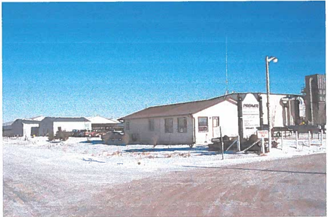
P.12 Office Building Looking North East
