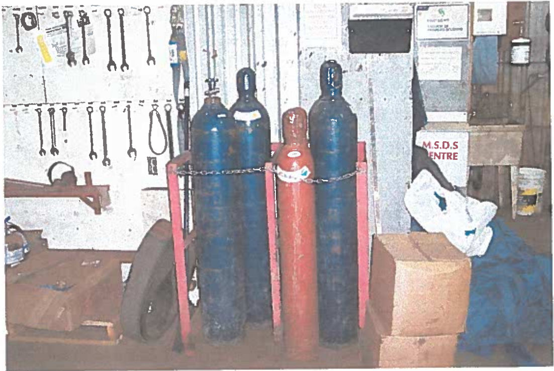
P.04 Welding Equipment Storage Area
