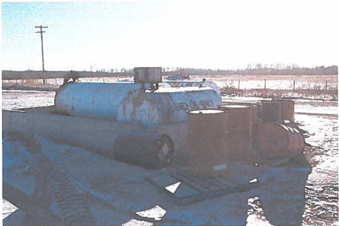
P.02 Used Oil Storage Tank And Concrete Crib
