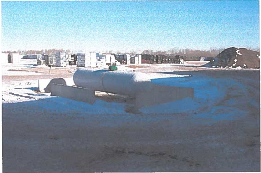
P.11 Another Propane Storage Area
