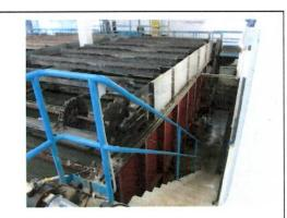
4.0 Removal of abandoned chemical feed systems and abandoned HVAC systems in the mechanical room.
