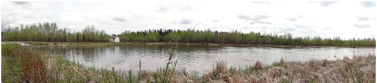
Figure 1.2: Existing Aerated Lagoon
