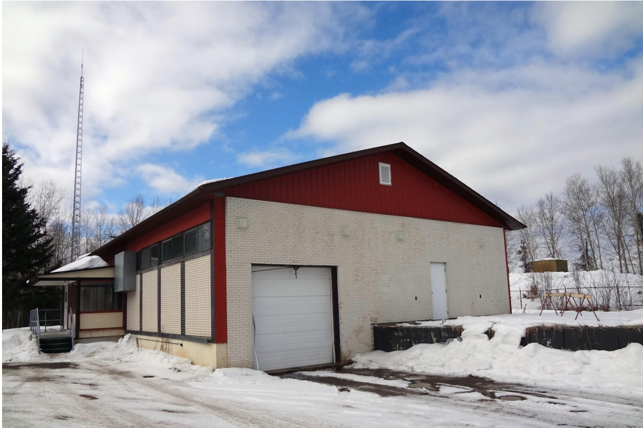
Figure 1.1: Existing Mechanical WWTP
