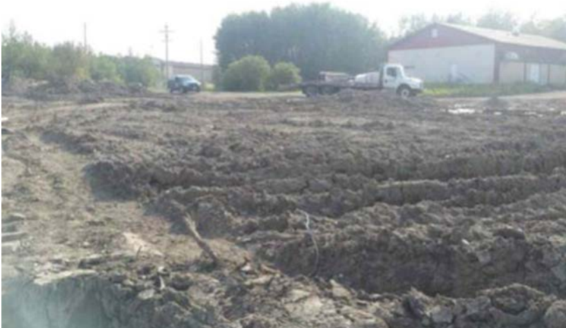
Figure 4.1: Clay Fill Exposed at the Surface of the WWTP Site
