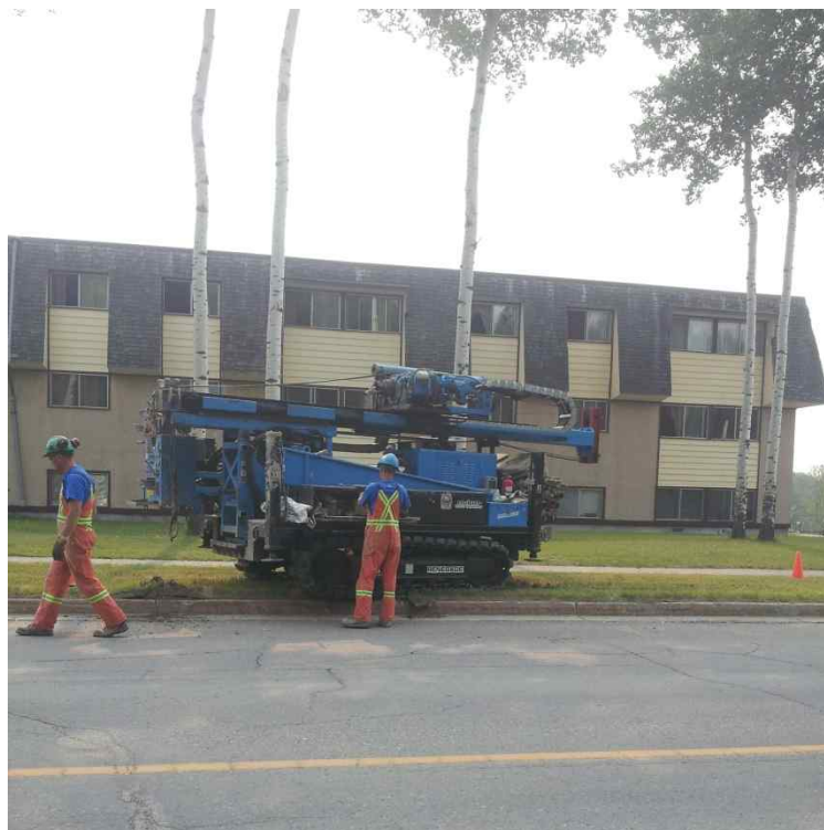
Photo 4 - Testhole TH11 drilled along proposed alignment for forcemain
