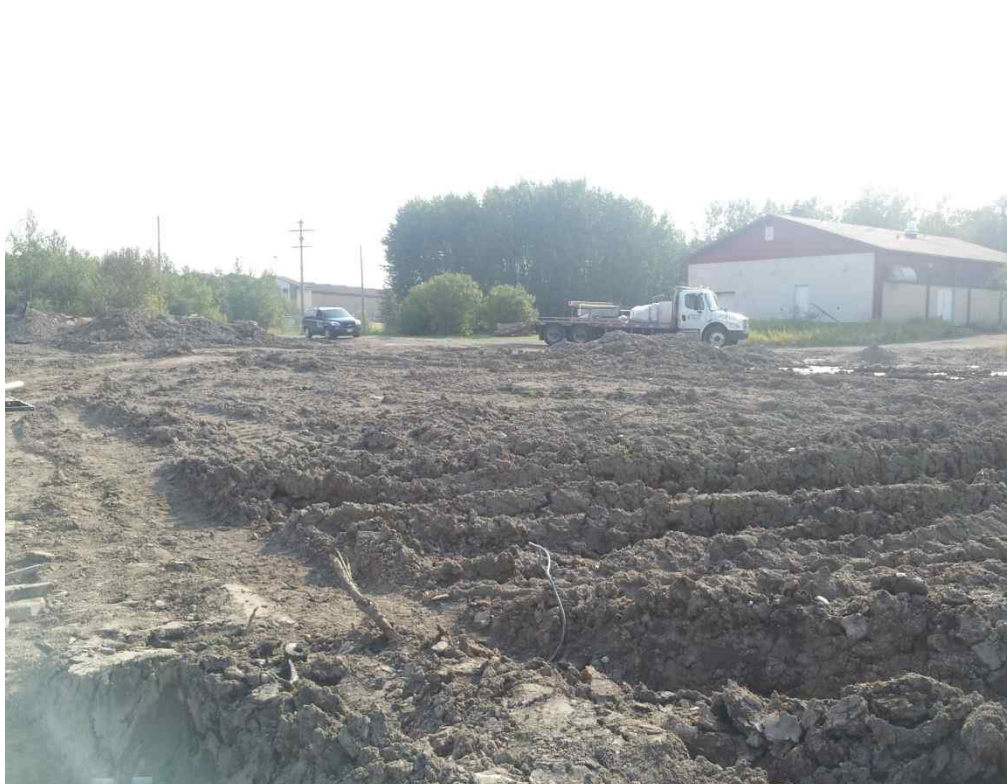
Photo 2 - Clay fill exposed at the surface of the WWTP project site
