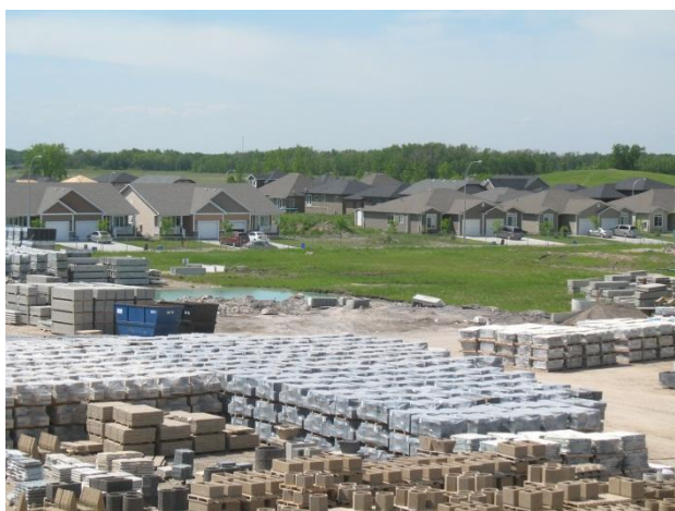
Photograph 11 ↑ Looking west towards proposed new paver plant location (06/13/13).
