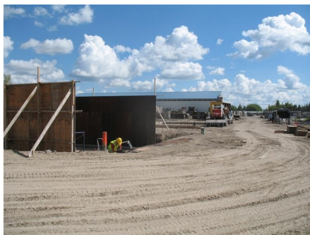
Photograph 12 ↑ Looking southeast at the construction of the rubble bunkers (08/01/13).
