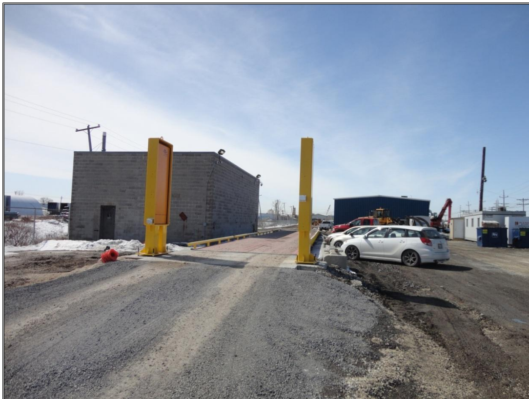
Figure 2: New weigh scale, radiation detector, and non-ferrous warehouse, looking west.
