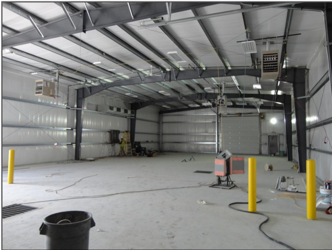
Figure 3: Interior of new building, looking west from the northeast entrance. This area will be used for indoor unloading of scrap by peddlers.
