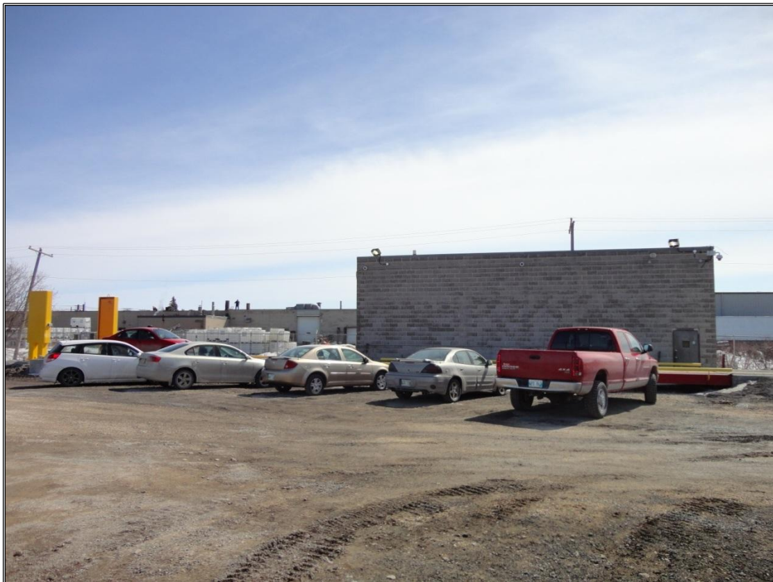
Figure 8: Alternate view of the non-ferrous warehouse that is used for storage of waste lead acid batteries, looking directly south.
