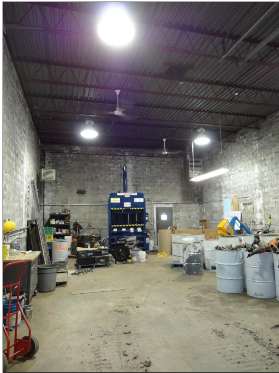
Figure 10: Expanded view of waste battery storage area inside the non-ferrous warehouse, looking east from the northwest entrance. Note the concrete flooring, concrete brick walls, metal roof, and sump pit.
