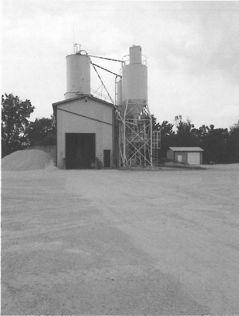
This is the batch plant. Some material such as fly ash is held in the holding tanks which you see above the plant.
