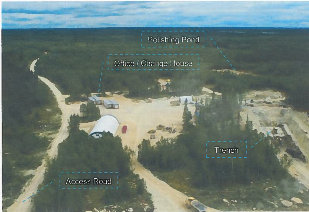
Photograph 1. Reed AEP Site under Development, looking east (August 2012) ↑
