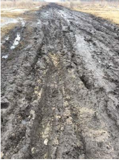
Figure 2: Beginning of Admixing
