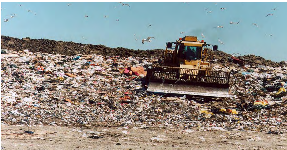
Photo 1-2: Typical working face and compaction equipment
