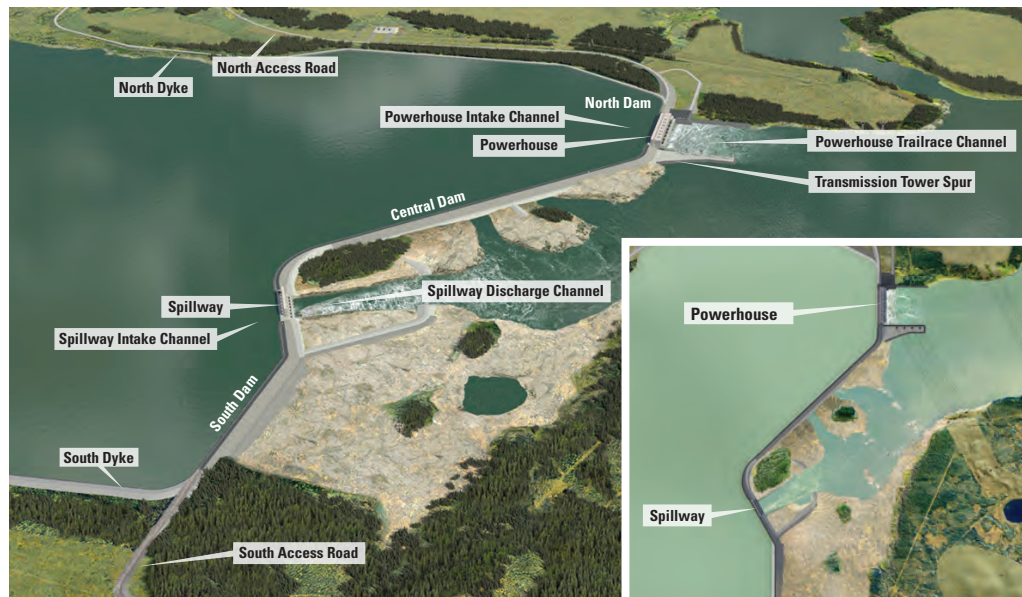
This rendering shows: the layout of principal structures at Gull Rapids looking north with the river flowing from left to right; how a portion of the south channel may look following construction dewatering and; the locations of the north and south access roads.
