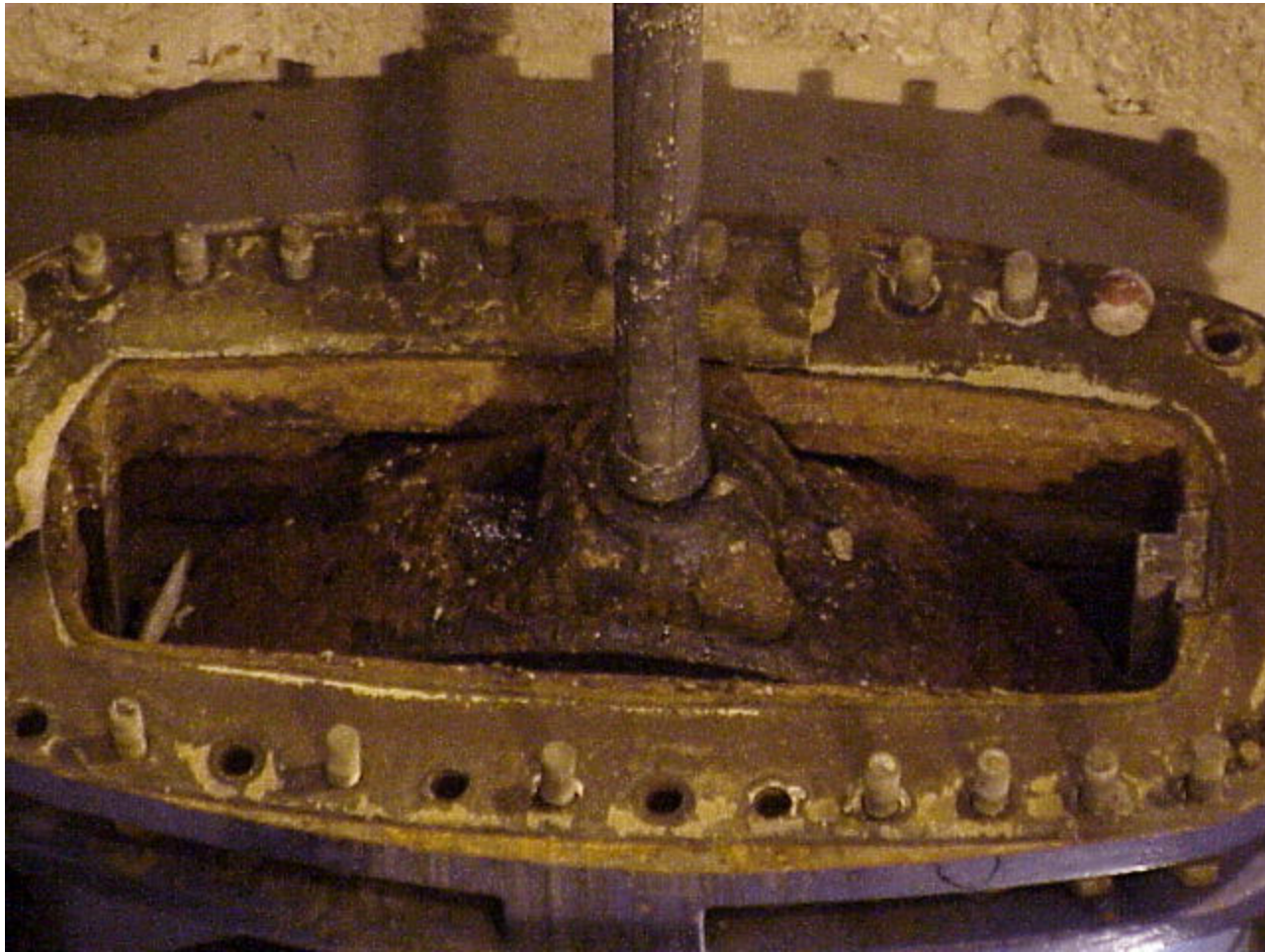
Viewing into the lower portion of the suction gate valve.
