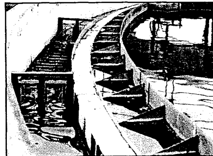
COPASACS REMOVING VISIBLE POLLUTANTS FROM FINAL EFFLUENT AT AN ACTIVATED SLUDGE PLANT
