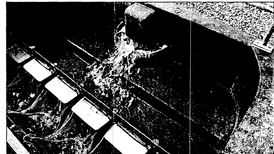
AGISAC ON EMERGENCY OVERFLOW AT A PUMPING STATION
