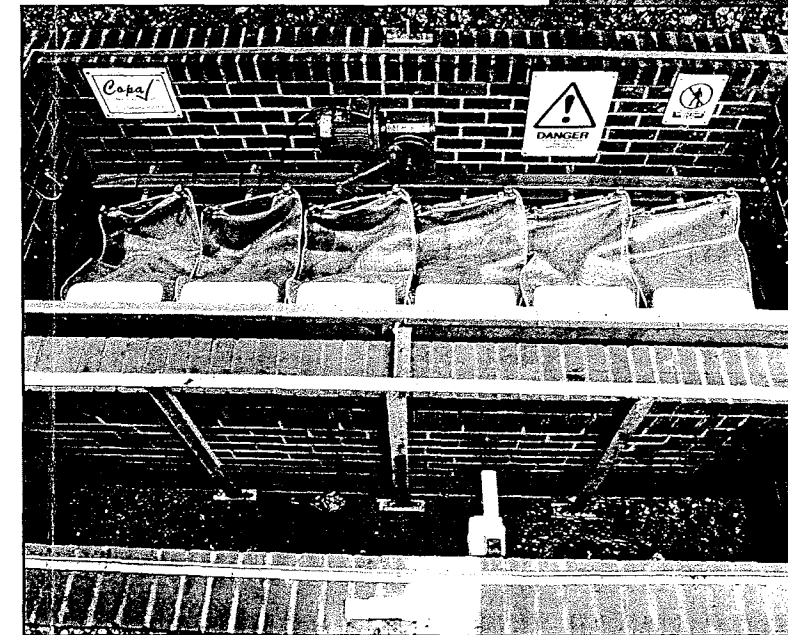
AGISAC ON EMERGENCY OVERFLOW AT A PUMPING STATION
