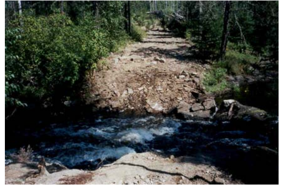
Stream banks reshaped following bridge removal
