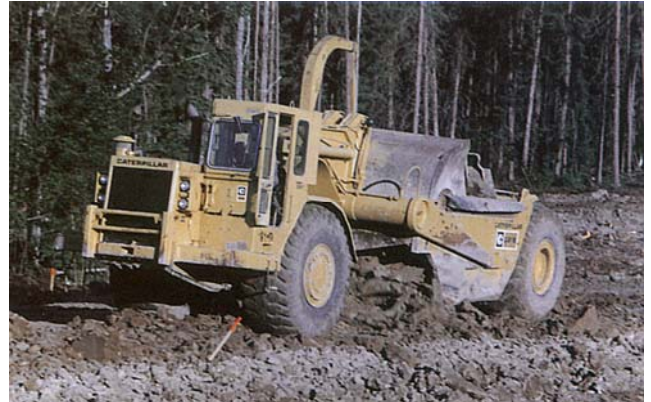
Scraper – combining ditching with fill for grade construction.
