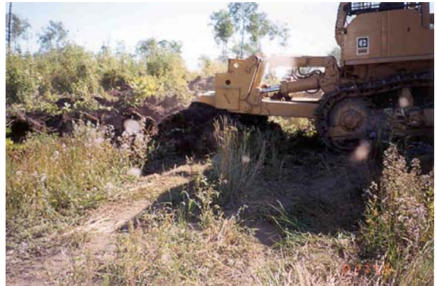
Tractor and V-plow treating right-of-way and road bed
