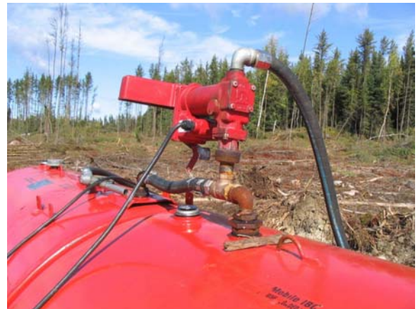
A nozzle not secured will result in fuel dripping on the ground and poses a higher risk of spillage
