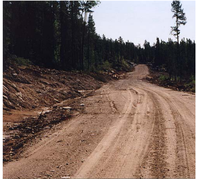
Drainage ditch along Class II Road.
