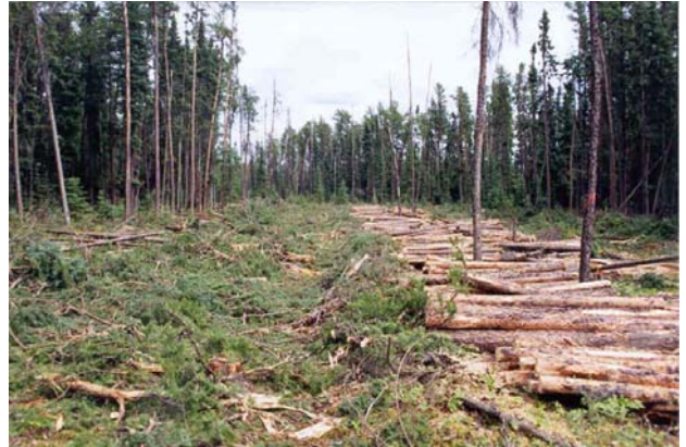
Winter clearing of road right of way
