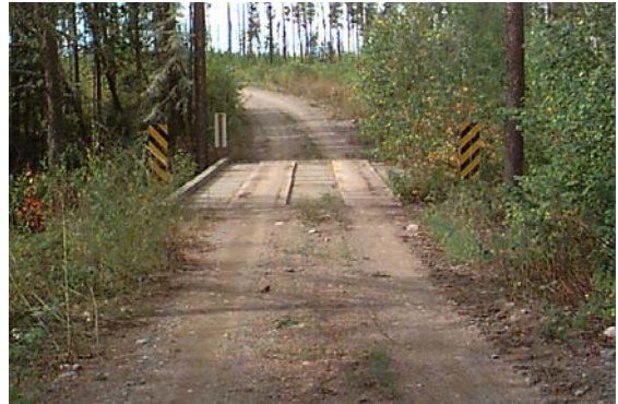
Minimal clearing for bridge approach
