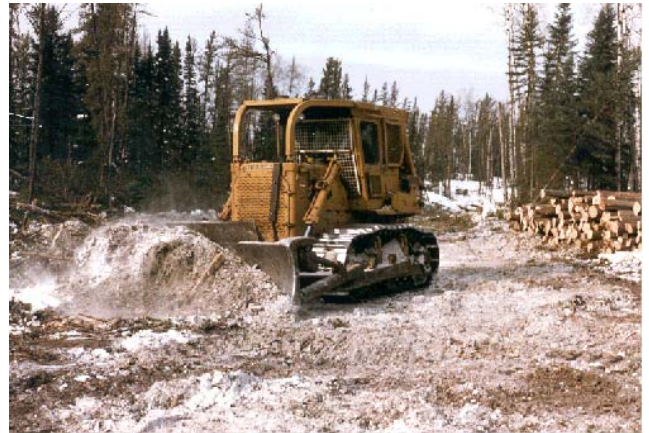
Levelling road surface
