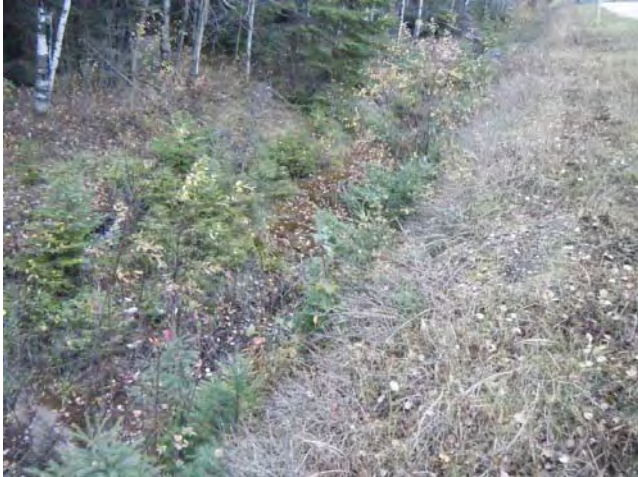
Photo 1. Typical view of PR 234 roadside ditch requiring a culvert for proposed access road.
