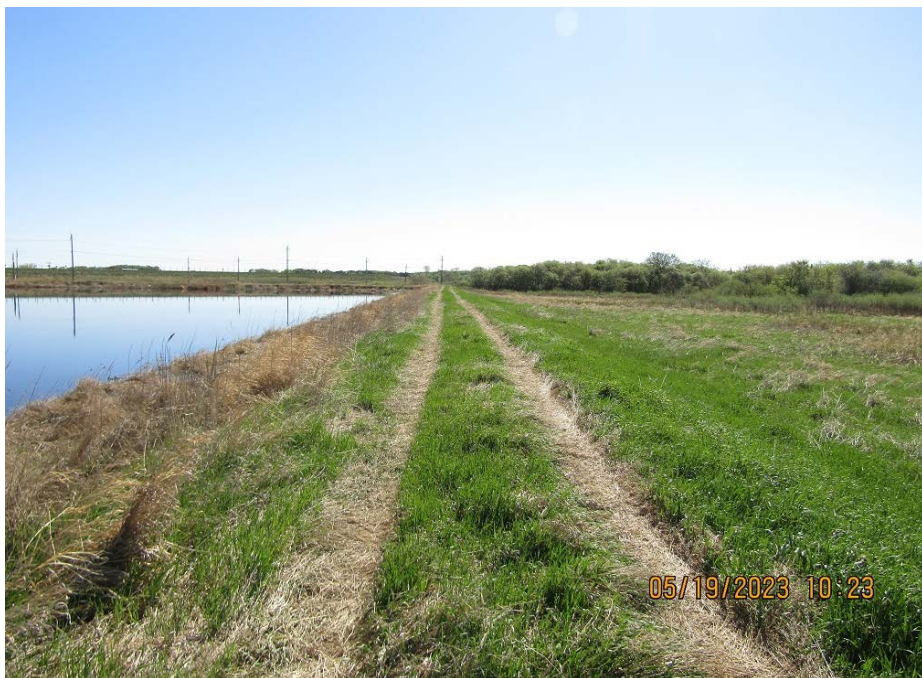
Berms in good shape
