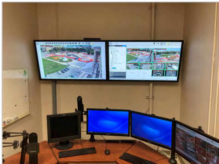
New Video Surveillance System Monitors
