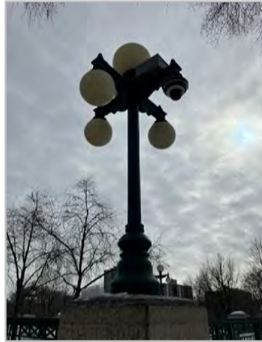
New Security Camera on an Existing Exterior Light Standard
