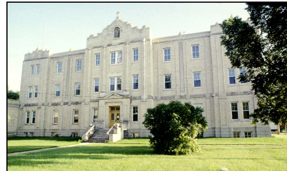
5.3.10 Above: Former Redemptorist Monastery
