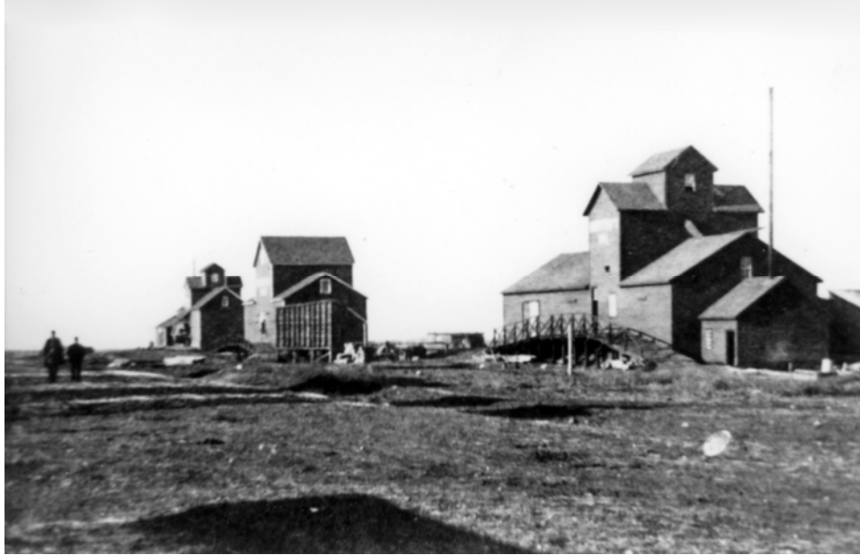
A row of early flat warehouses in Virden, c.1885. It is interesting to note that even at this early stage, all of these structures had already been enlarged, or were in the process of being expanded. (PAM)
