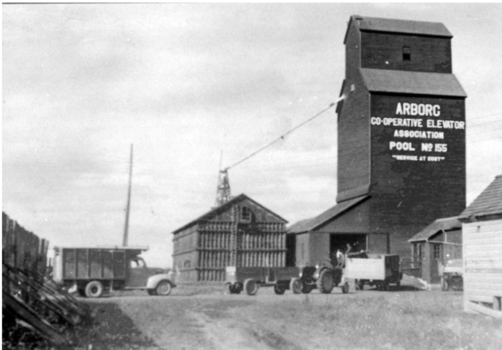
The Arborg Co-operative Elevator Association, Pool No. 155, c.1960. Note the unusual location of the 1940s style Overgaard annex, in this case positioned to the side, rather than in front or at back, of the main structure. (PAM)
