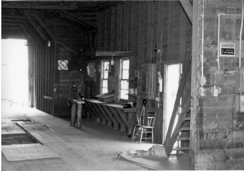
A typical elevator driveway. The receiving-pit grate can be seen at left and the platform-scale balance-beam at centre. The doorway on the right leads to the elevator office, accessed via an open walkway. (Inglis 245.L.2)
