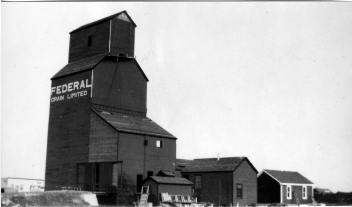
Construction of the Federal Grain Company elevator at Broad Valley c.1939. By this date, all elevators being constructed had tall entrance driveways to permit the unloading of grain from farm trucks fitted with hydraulic box hoists. Note also the presence of several small storage buildings adjacent to the office. (M. Roche photo)
