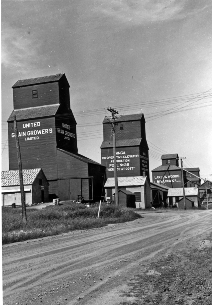
A row of five elevators at Ninga, three standard plans and one pyramidal. When photographed in 1955, all were in excellent condition. None of these structures have survived. (PAM)
