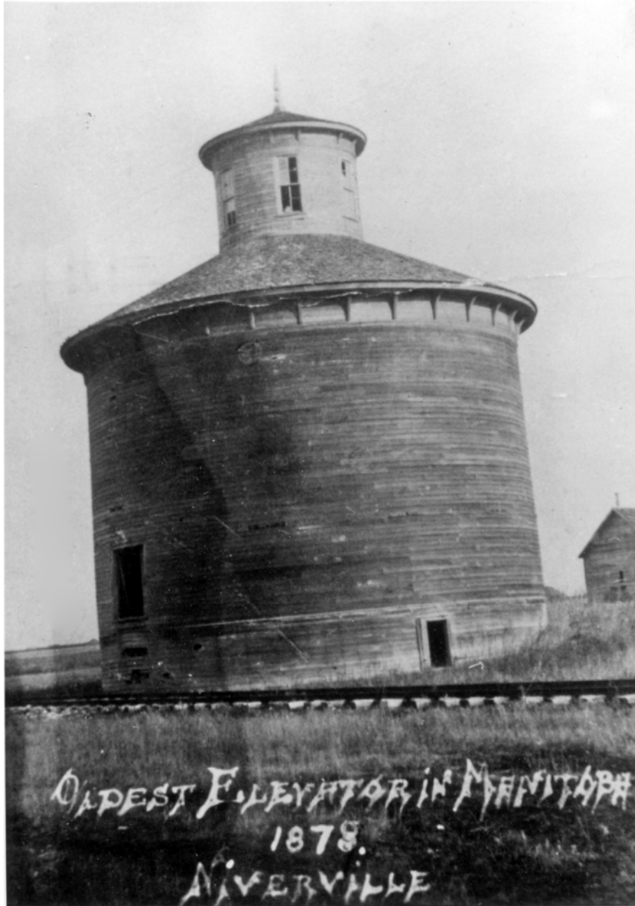
Constructed in 1878 in Niverville, this unusual structure was western Canada's first commercial grain elevator. In operation until 1904, it had a capacity of 25 000 bu. And featured horse-powered grain-handling equipment. Photo c.1911. (PAM)
