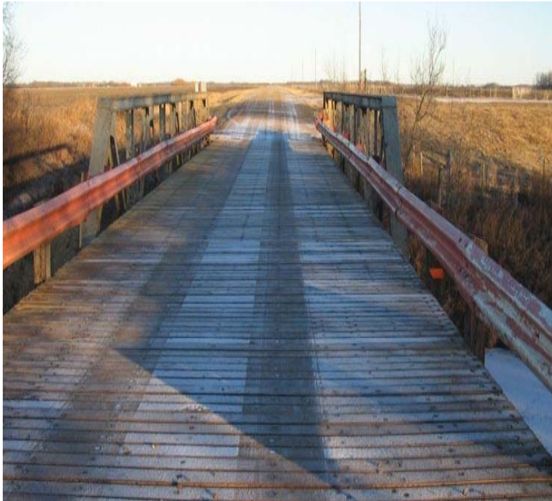
RM of Dauphin - Henderson Bridge
